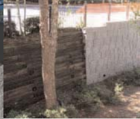
▲ The timbers facing the wall below a tennis court had failed. The owner wanted the wall repaired while the tennis court was in use. By using the Landmark system, the wall was refaced, and play was uninterrupted.
