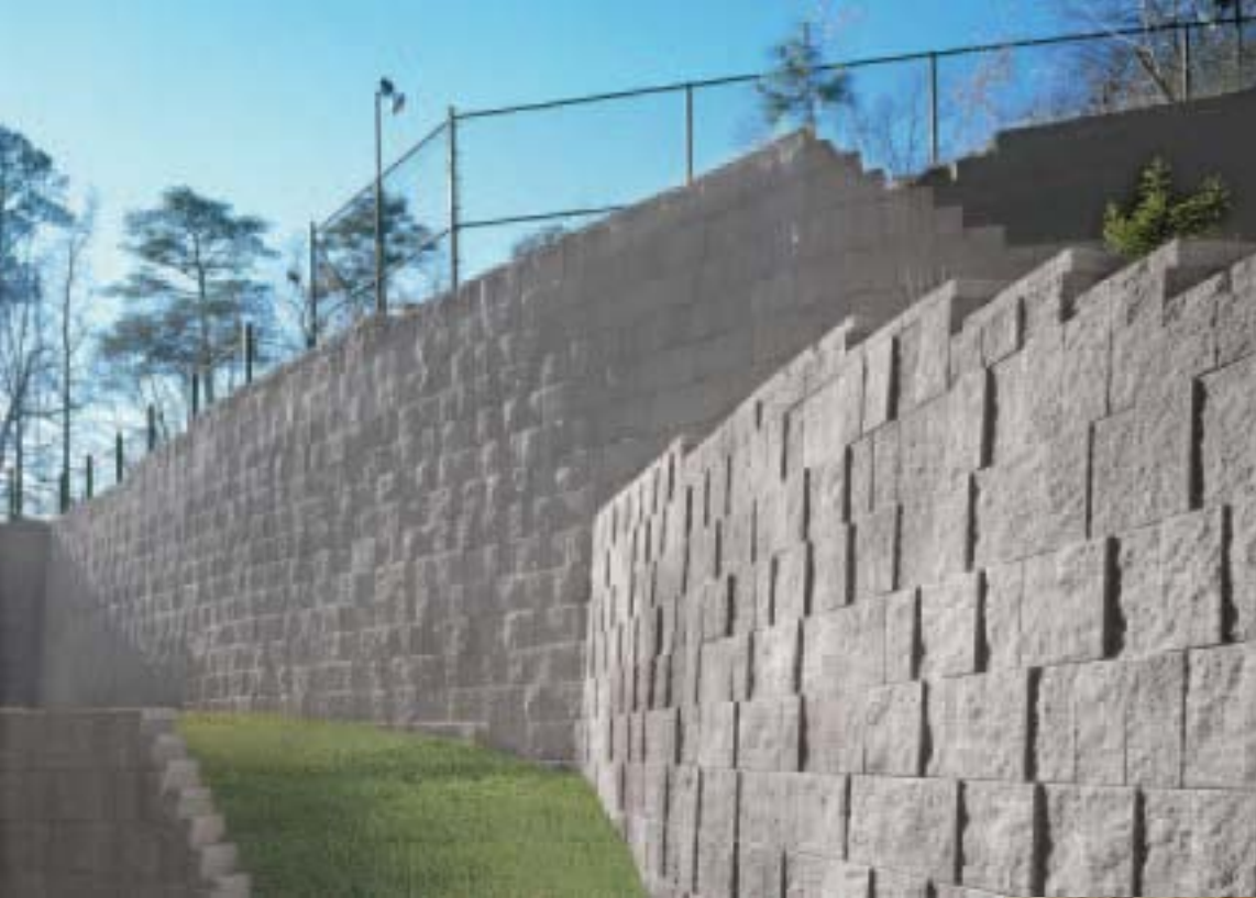
▲ The timbers facing the wall below a tennis court had failed. The owner wanted the wall repaired while the tennis court was in use. By using the Landmark system, the wall was refaced, and play was uninterrupted.
