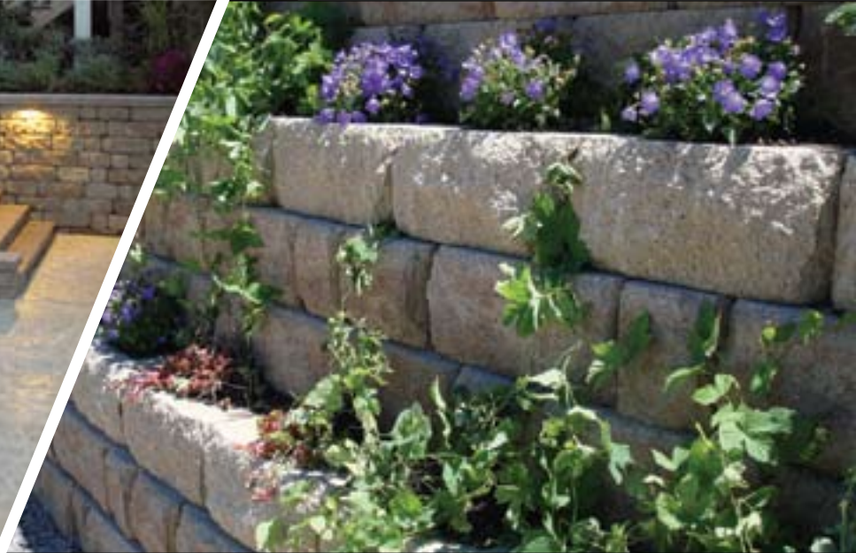
PLANTER BLOCK RETAINING WALL
